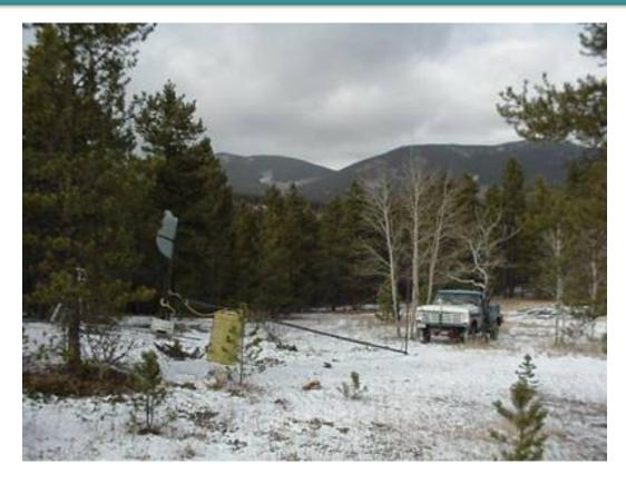
The windmill ready to be raised...everything looks A-OK. The mast is 35 feet high with 3" steel pipe at the base, and a 1 1/2" pipe jin pole with a brace welded to the bottom. The windmill has an 8 foot 3-bladed rotor, powering our homemade permanent magnet alternator (in tests, 60 amps in 40 mph winds!).
