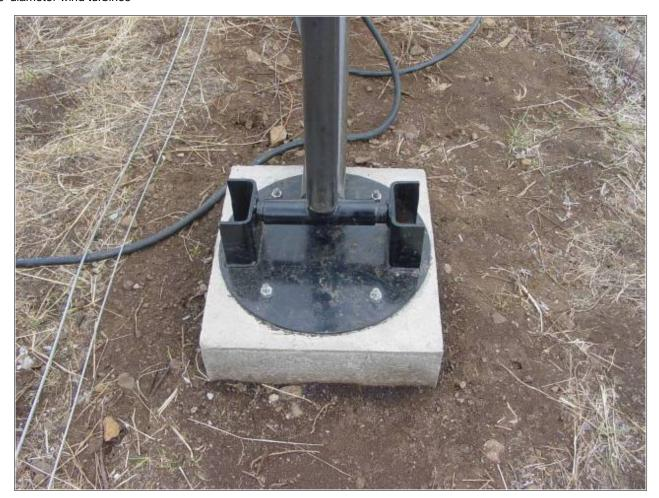
Above is pictured the hinge for Georges tower. The tower is 41' tall. When we made the hinge, we welded pipes to the hinge so that the gin pole and the tower itself could simply slip over these pipes, and we could hopefully assemble it on site with no welding.
