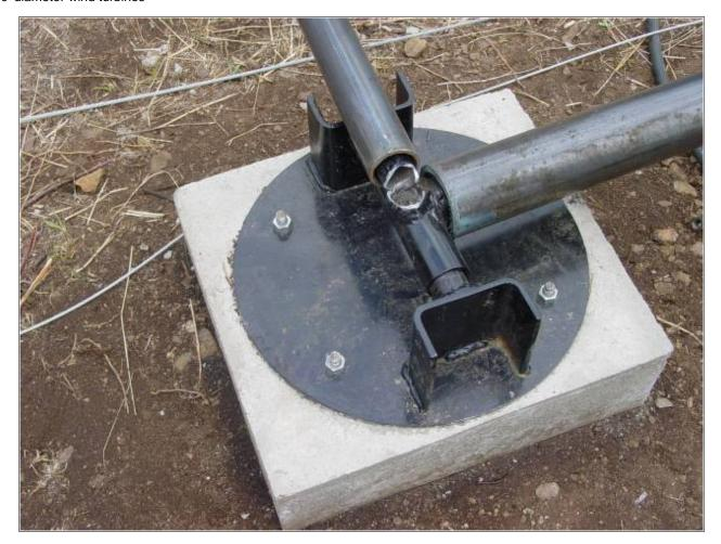
We went to raise her with a truck. Got the windturbine about 10' off the ground when the jin pole snapped off! Normally we'd put a gusset in to strengthen things, but we figured it'd be strong enough.. and this simplified the on site assembly (so we thought). It probably cracked when we test raised the tower, and it came past center to rest on the jin pole before we had the guy wires adjusted properly. Basicly.. it simply wasn't strong enough. Lesson learned!
