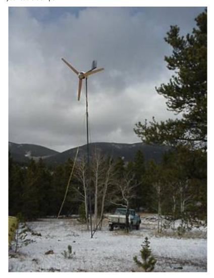
We just about got it up! Note that the end of the jin pole bent from the stress, but held on past its point of maximum stress, enough to get things vertical. Everything appears to be going good, BUT SOMBODY FORGOT TO TIGHTEN THE CABLE CLAMPS ON ONE THE SIDE GUY WIRES. Everything tilted hard to the side opposite the unfastened guy wire, and the mill came crashing to the ground. No injuries to humans, dogs or trucks.
