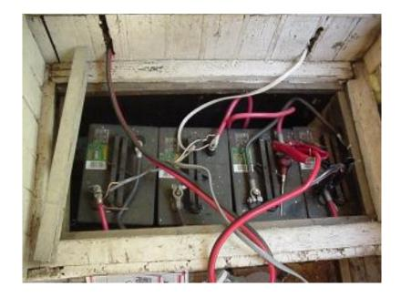
The battery bank, with 4 golf cart batteries. Can anyone spot the safety hazard here? (sorry Dave, couldn't resist...) It has to do with the awl and the jumper cable clamps that connect to the inverter! He's fixed it by now I bet.
