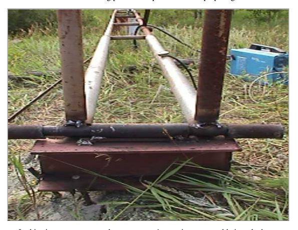
In this picture you can see the tower as we're starting to assemble it to the base.
