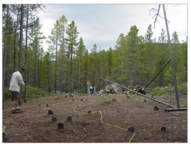
Here is the tower on the ground. It's 43' tall, from 3" diameter pipe. The top 10' are reinforced -hopefully it's rigid enough. The base is a simple pivot which is staked to the ground, and all the guy wire mounts are drilled into rock nearby. At 43', it gets nicely above the trees looking to the North, West, and South - but to the East its not high enough. The prevaling wind here is from the West so it should workout OK.
