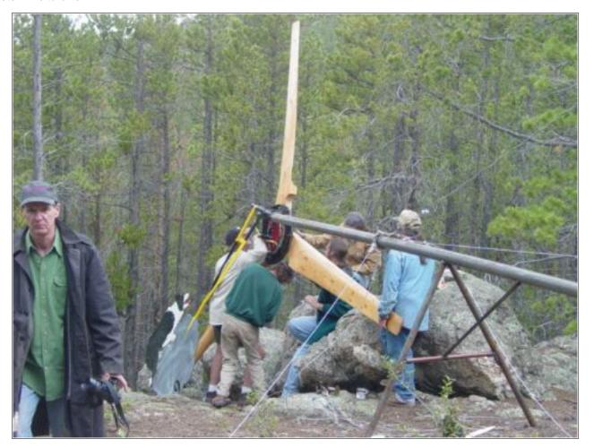
Pictured above neighbors are helping to assemble the machine on the tower top. You can see I've welded a support, or 'Foot' on the tower so that when the machine comes down the tower is not able to hit the ground. This makes it a bit easier and safer to work on.
