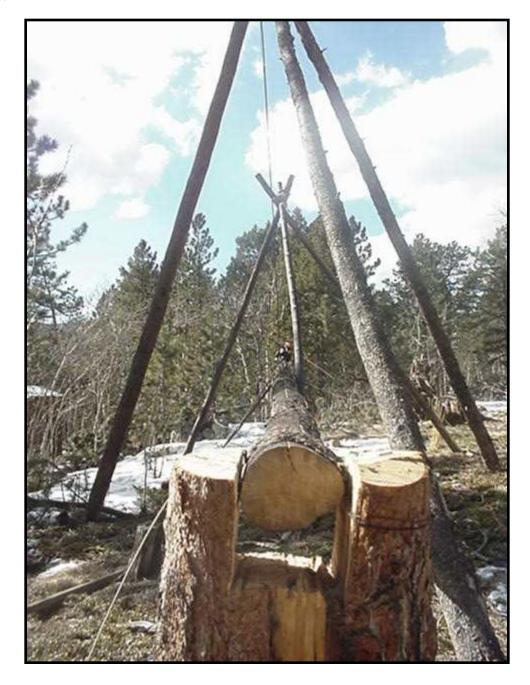
I simply used a truck, a long cable, and the large tripod to raise the mast, it went smoothly!
