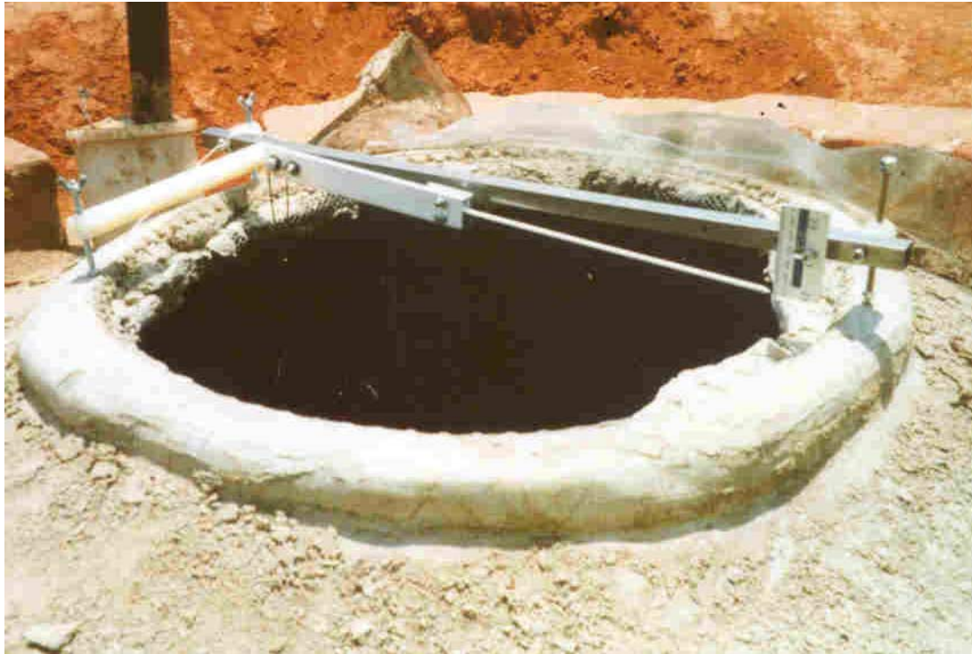
Figure 4 – Leakage test apparatus being tested in the field on a PBG tank
