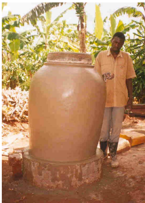
Figure 9 - 400 litre water storage jars being constructed as part of the water quality testing experiments in Uganda
