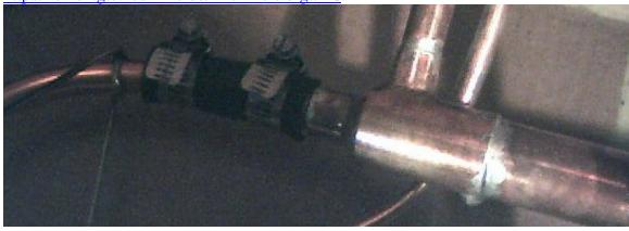
Deburring of the ridge inside the .5" end of the copper T is necessary for the .5" pipe to slide all the way though to the other end. This can be done with a round file or a rotary rasp on a drill
