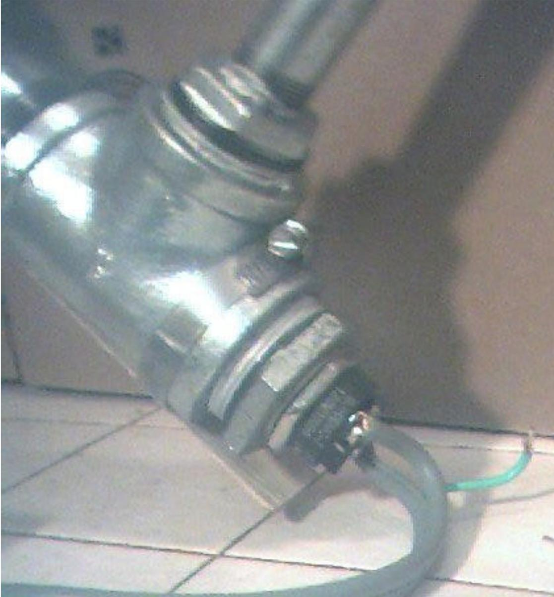
This is what the heater element fully installed looks like and with a wood strip held on with a hose clamp for bump protection. The ground wire is put under the hose clamp to ground the pipe assembly.
