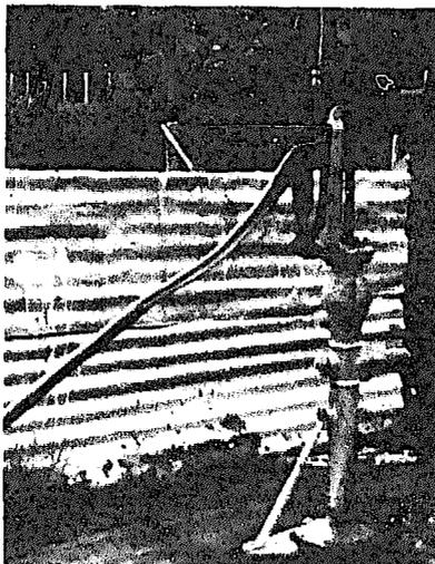
The below ground components of the DMR Dempster derivative are conventional and required the usual repairs to worn leather cupseals, footvalves and leaking joints. The threaded connection between the pump body and the 1-1/2 inch diameter galvanized steel rising main proved especially prone to fatigue failure.
