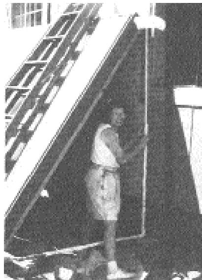
Ilene wraps the plastic pipe so the sun won't degrade it.
