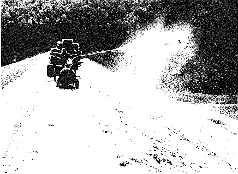
Fig. 13-12. Mulching machine operating on new fill.
