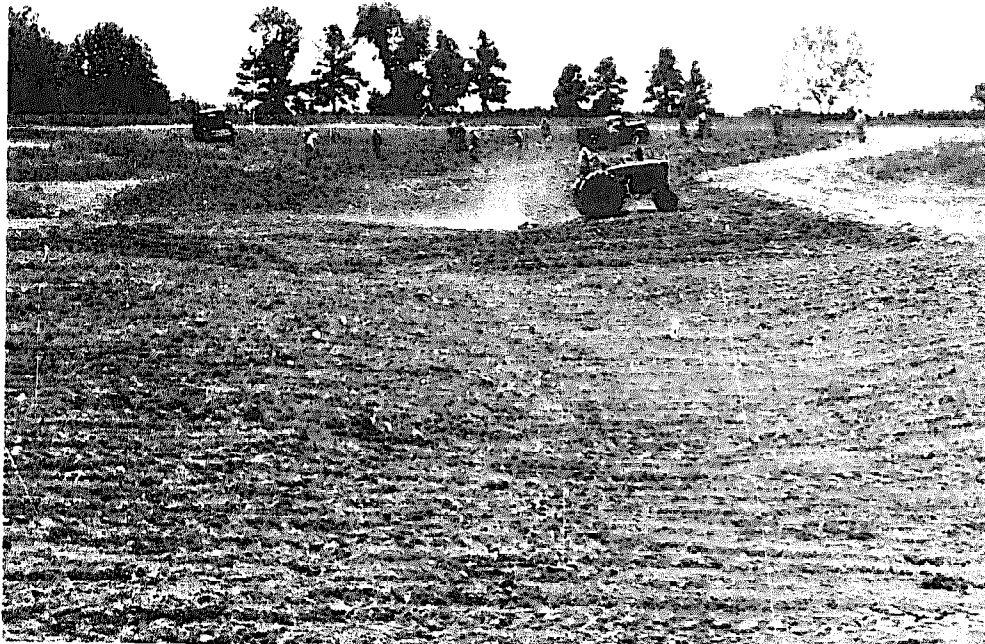
Fig. 12-2. These two pictures show how a gullied area is turned into a useful waterway.
