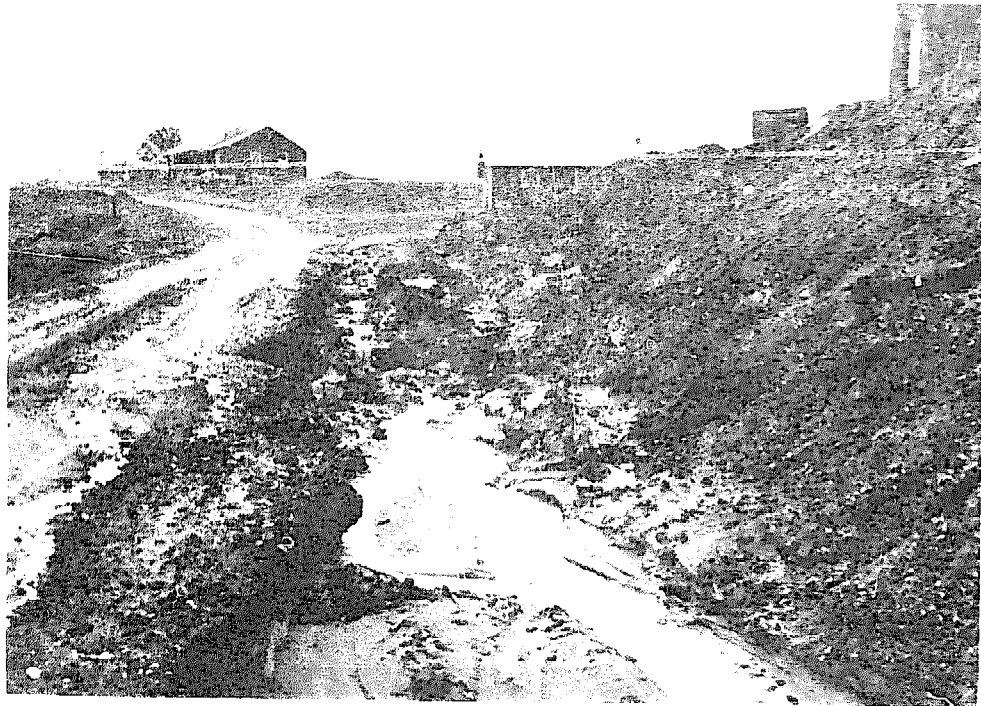
Fig. 13-1. Uncontrolled runoff damages the construction site and carries the sediment that damages areas downstream.
