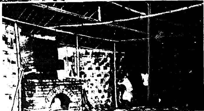
8. View of interior of partially completed building.
