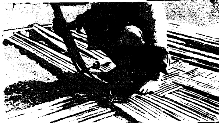
3. Fabricating walling from split bamboo.
