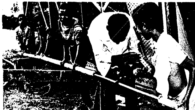
2. The drilling operation
