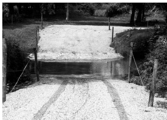
Figure 1. Full Stream Crossing
