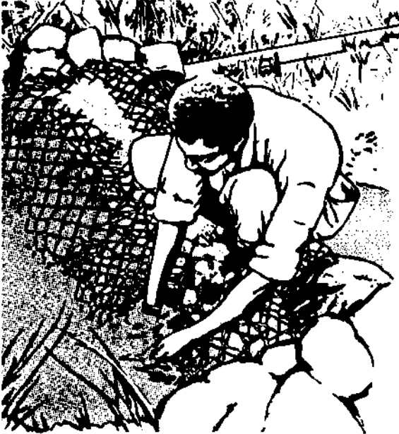
Building a gabion dam
