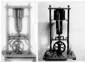
**1832 ~ ROTARY DC GENERATOR (COMMUTATED DC GENERATOR)**
