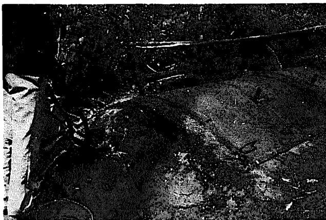
During the lighting stage, seal the edges of the overlapping joints of the metal cover with soil. Apply soil also to the edges of the metal sheets overlapping the mud walls at each end of the kiln and along the sides of the kiln where the cover is held in place by the angle-iron framework.
