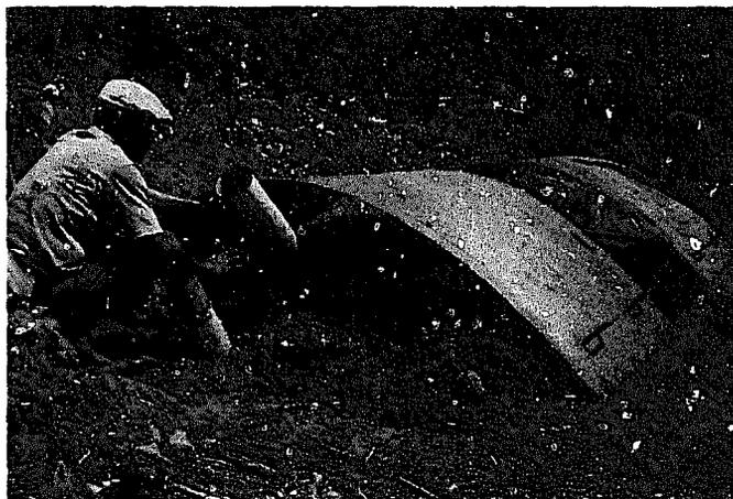
The final construction of the end walls of the kiln is achieved by the builder plastering with mud from inside the kiln.
