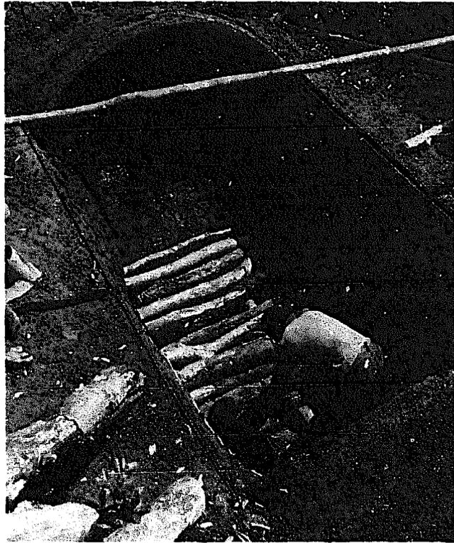
Load the remainder of the wood making sure that the larger diameter billets are placed in the centre of the kiln. Fill in the sides of the kiln and any holes between the larger billets with smaller wood so that the maximum amount of wood is packed in.
