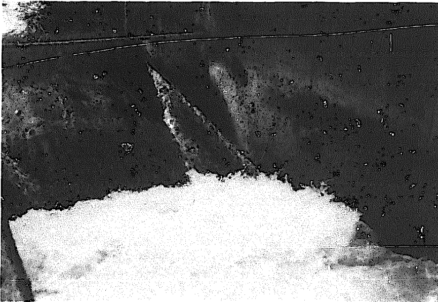
Figure 13.6. Hydraulic jump for rapid mixing (Philippines)
