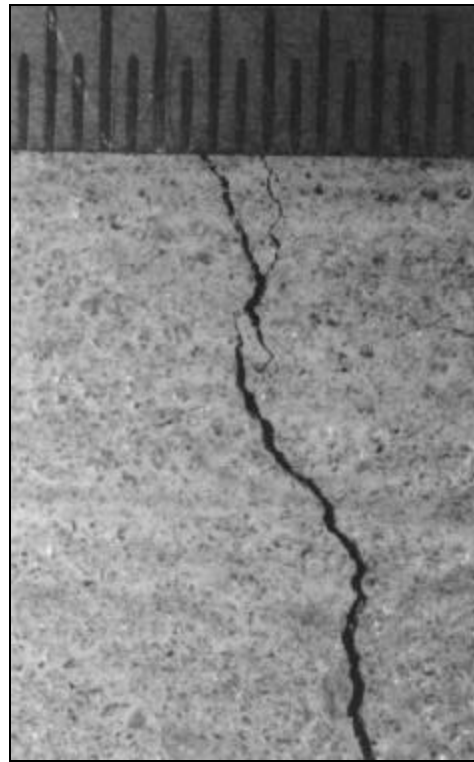
Fig. 5.21(b) Large cracks in chicken wire reinforced specimen
