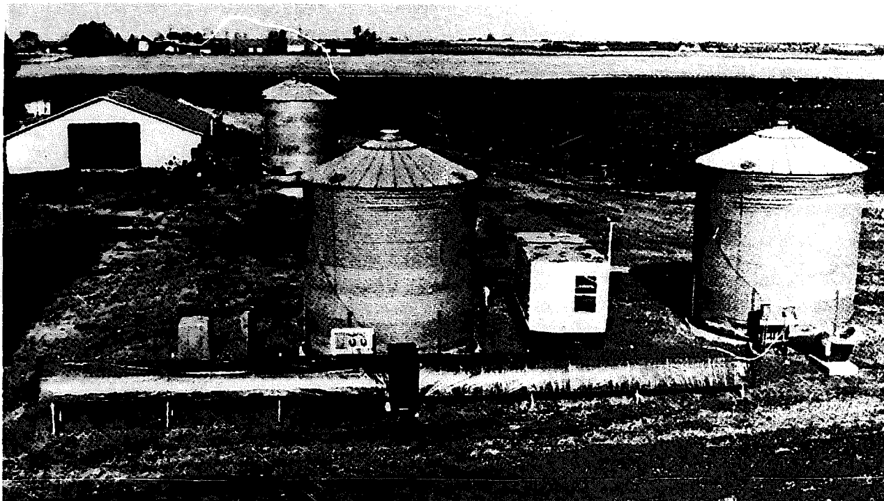
Figure 5 Stationary Suspended Plate Solar System used in corn drying experiment. Location: Iowa Agricultural Experiment Station, Ames, Iowa
