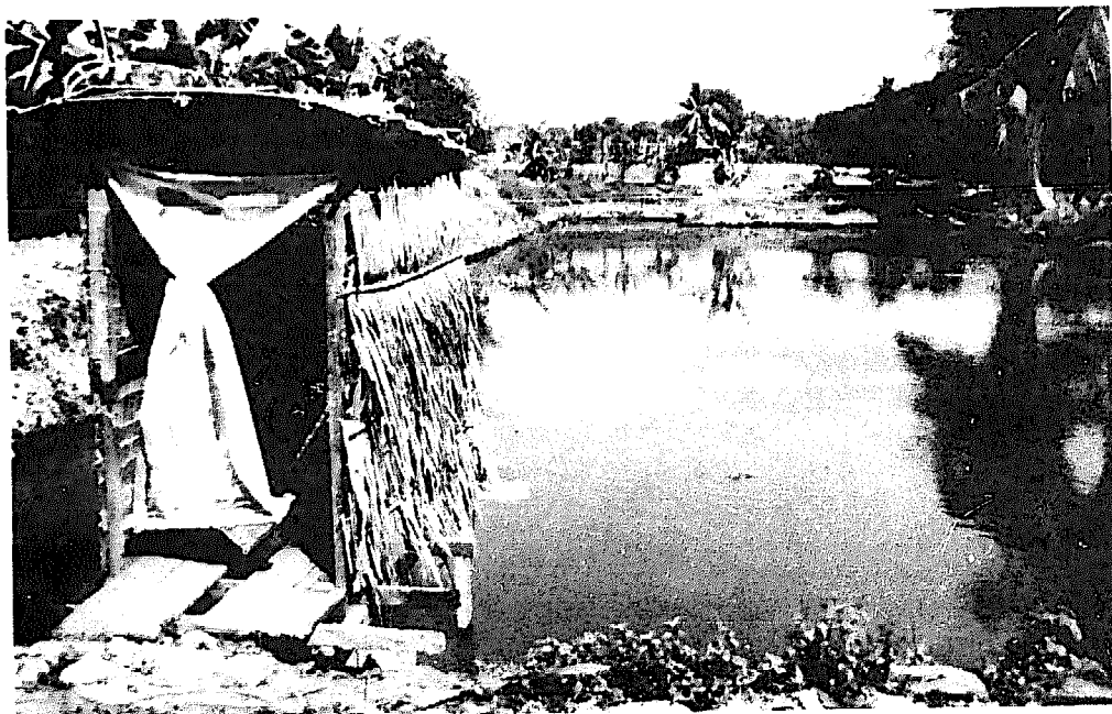
Fig. 2 Overhanging latrine on fish pond, Pathumthani, Thailand.
