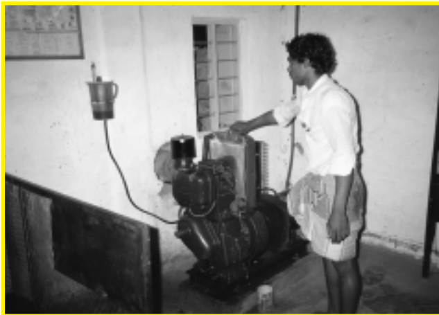
Street lamp lit by biogas-derived electricity (top). Biogas and engine electricity generator with operator in village of Pura, Karnataka State, India (bottom).
