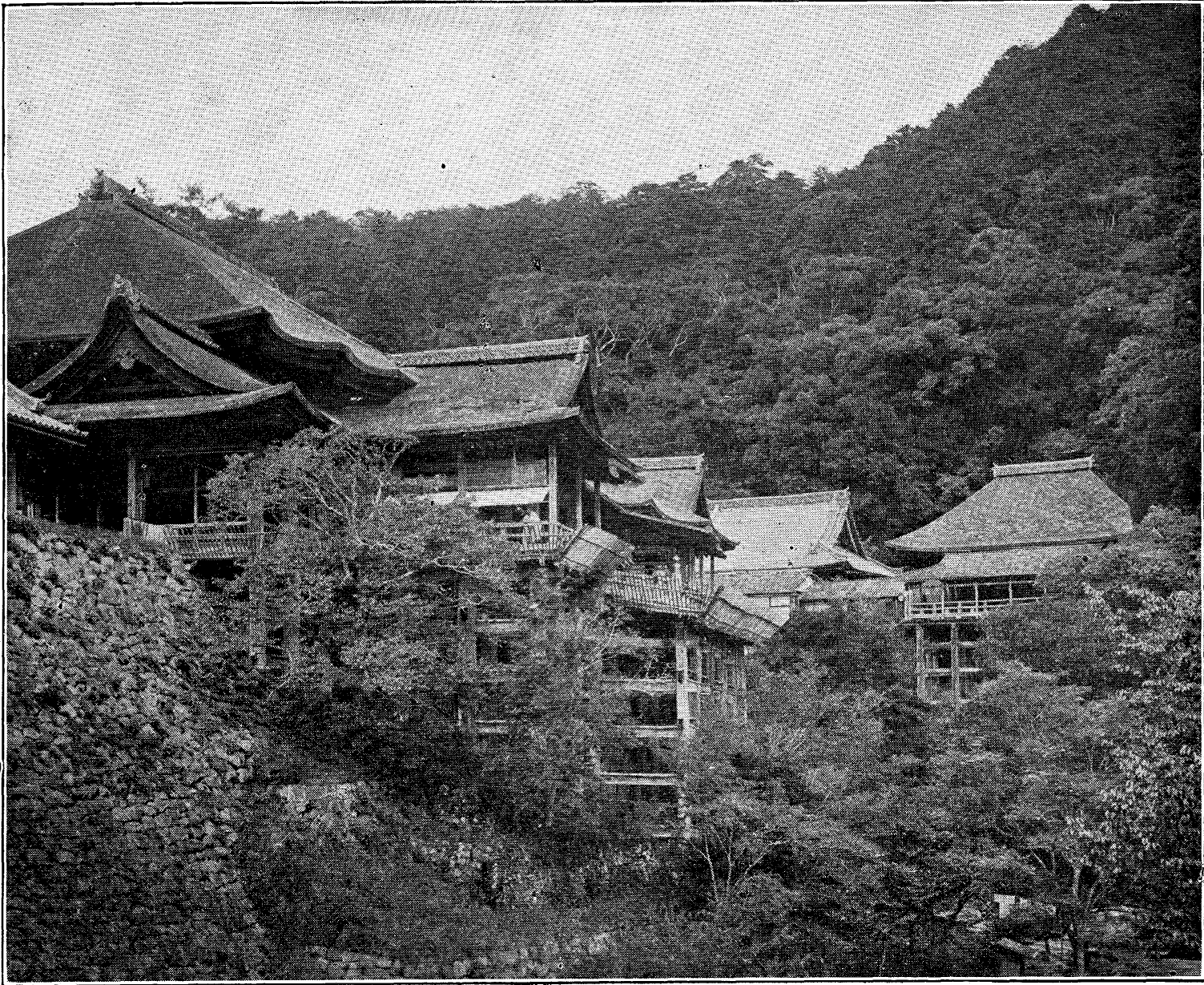
Fig. 236.—View of Kiyomizu temple and the wooded mountain slope rising beyond, showing how dense the forest growth may become when long protected.
