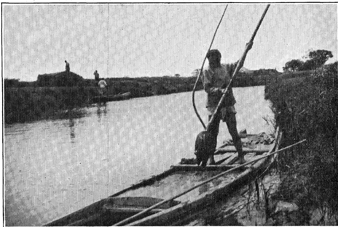
Fig. 103.—The young man is loading his boat with canal mud, using the long-handled clam-shell dredge which he can open and close at will.
