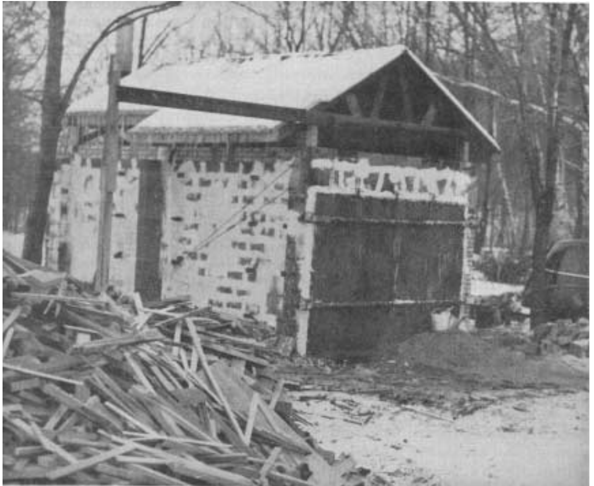
Figure 15. --Experimental single-wall, masonry block kiln.
