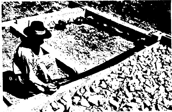
Fig. 55 Damp course of bituminous felt.
