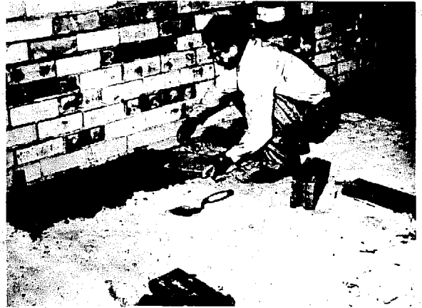
Fig. 86 Laying floor tiles.
