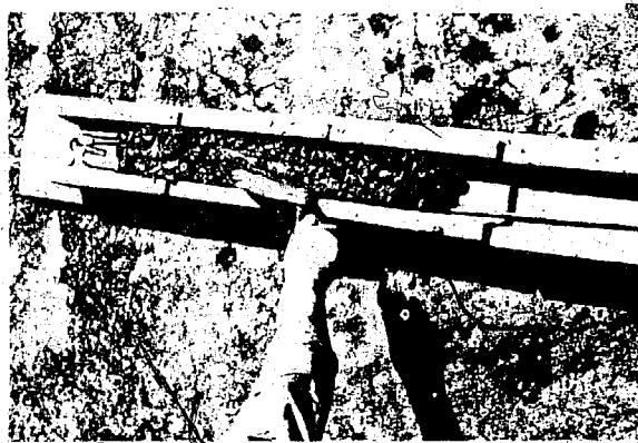
Fig. 68 Lintel prefabricated in U-blocks.
