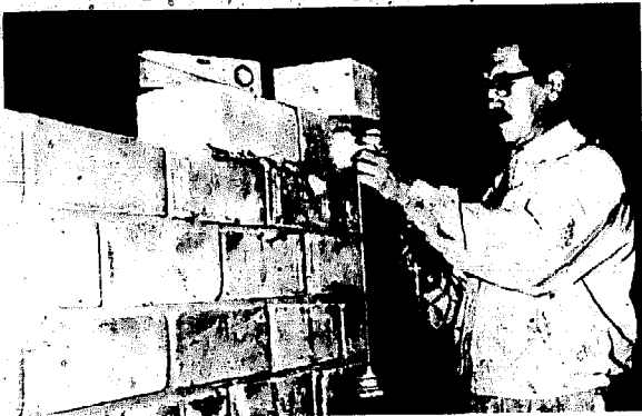
Fig. 56 Building a wall of soil-cement blocks.
