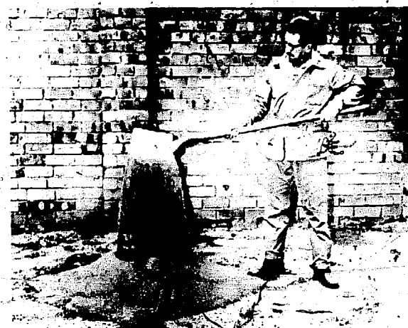
Fig. 26 Adding cement to the soil.
